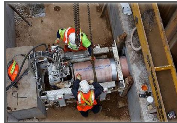
Auger Boring / Pipe Jacking
