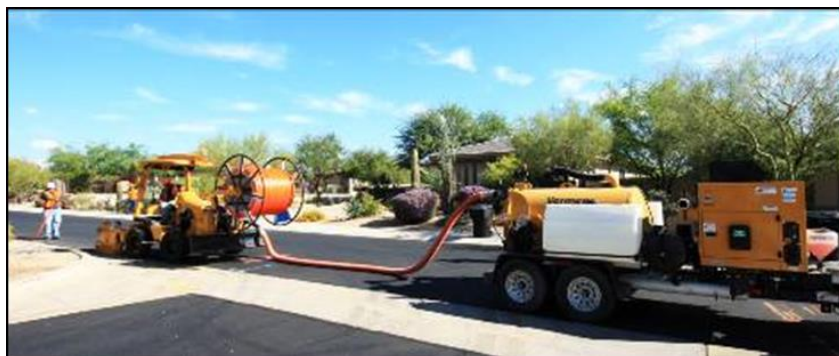
Micro-Trenching with Vacuum Excavation
